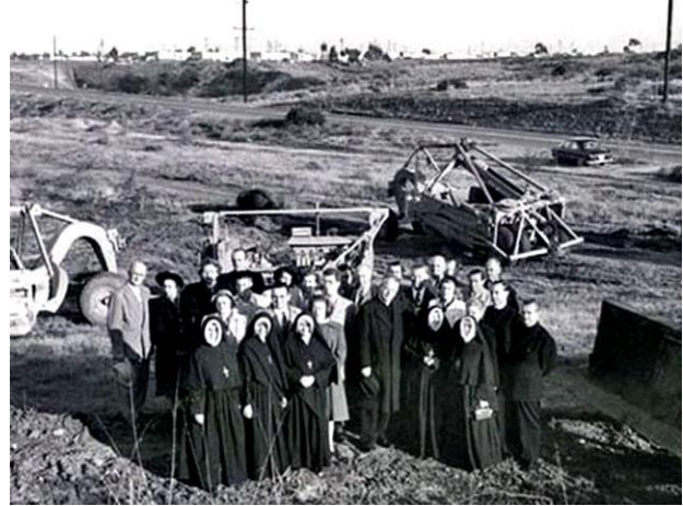
Bulldozing for the Construction of the San Diego College for Women Note the Presence of Five Sacred Heart Sisters
